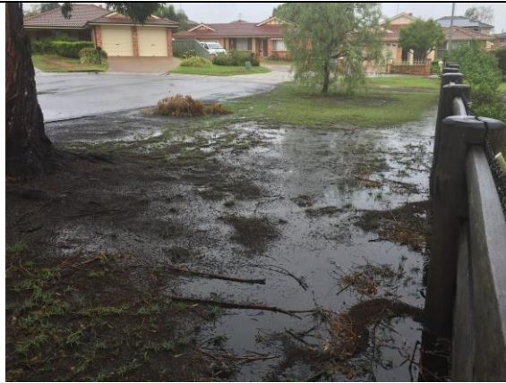
Plate C4.1 – Floodwater ponding between road and front of properties that are located on the western side of Linden Crescent, Cranebrook.
