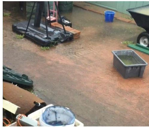
Plate C5.6 – (Photo taken at 13:30 hours) Floodwater ponding at rear of property that is located on Linden Crescent, Cranebrook.
