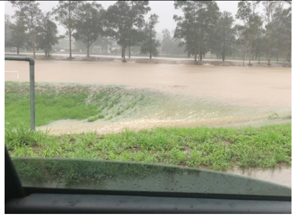
Plate C5.2 – (Photo taken at 15:00 hours) Floodwater surcharging the spillway of the Borrowdale Road Basin No. 2.
