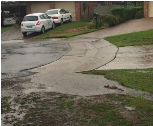
Plate C5.5 – (Photo taken at 10:00 hours) Concentrated flow discharging from gutter in Linden Crescent, Cranebrook.
