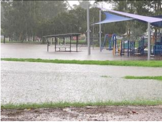
Plate C5.1 – (Photo taken at 12:00 hours) Floodwater ponding in the Borrowdale Way Basin No. 1.
