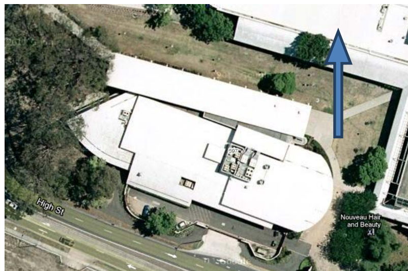
Figure 15: Aerial view of JSPAC showing large northern aspect
